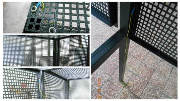
Please use the special edgy spacers when fastening each end of the grounding cables. Their function is to ensure the metallic contact on the painted surfaces to provide the equipotential connection of every metal part as well.
